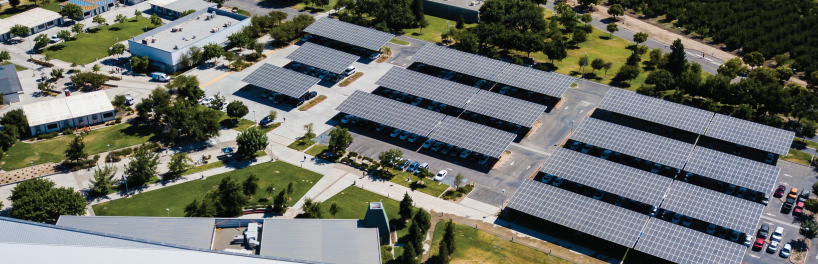
888 kW solar parking canopy system for Madera Community College Center by member company, ForeFront Power, as part of a 7.4 MW portfolio for State Center Community College District.
